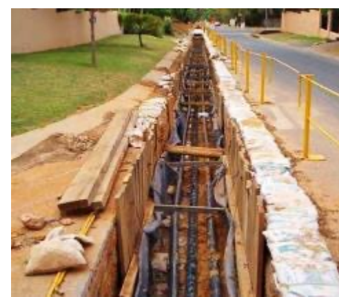
Integrated utility relocation
