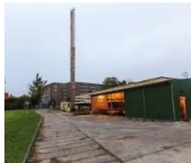
AgroTherm GmbH (Malchin, Germany): 800 kW boiler using fen biomass from paludiculture for district heating. More info: BOnaMoor project
