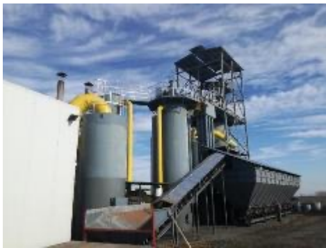
Vioenergiaki Patridas (Veria, Greece): 1 MWe gasifier using wood chips from peach tree plantation removals. Image source: M. Karampinis
